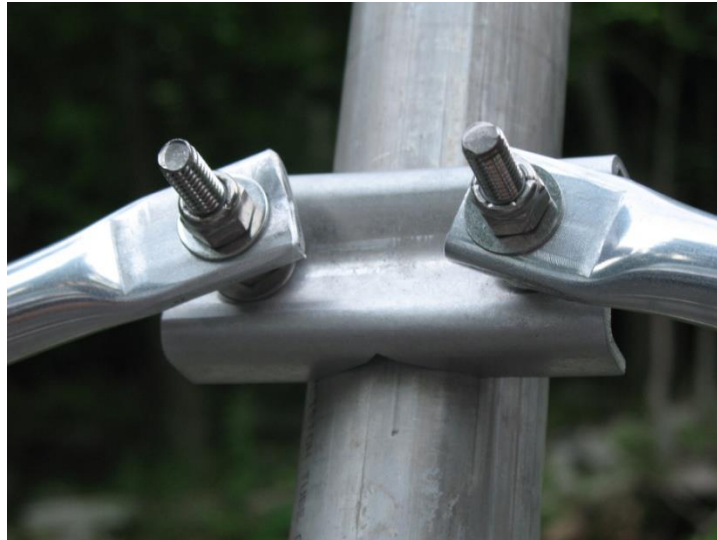
Photo 3: Mast Truss Support
