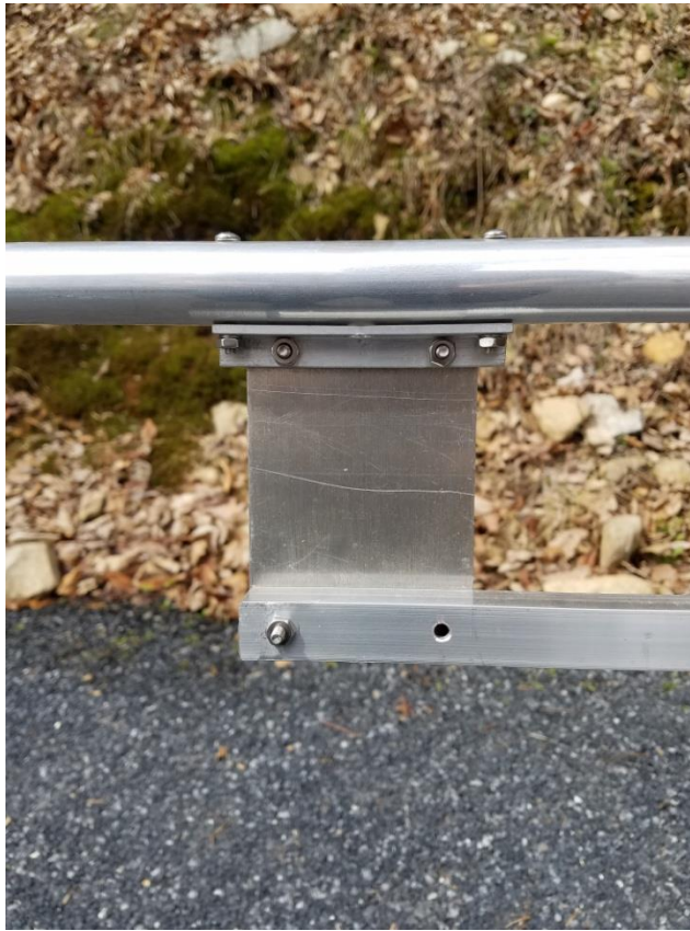
Photo 2: Sub Boom Bracket and Plate
